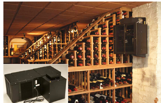
Freestanding Wine Guardian Humidifier (above) Integrated humidifier on ductable system (left)
