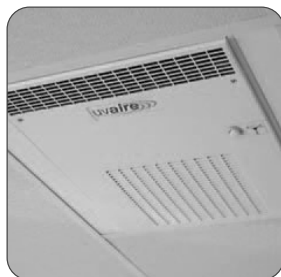
Drop ceiling installation (side panels adapt unit to fit standard 2' x 2' grid)
